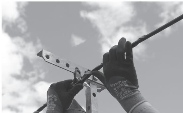
4. Insert the device into the crossarm, by alignment of the holes in the cap with the hole in the crossarm (as in the pictures below).
